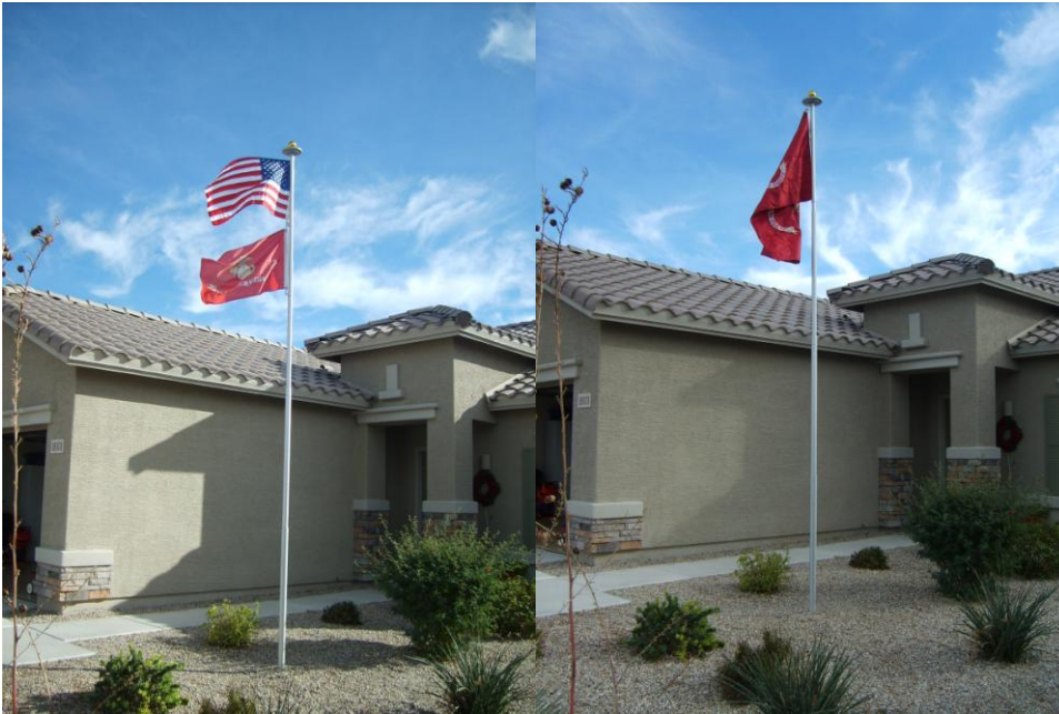
Telescoping Aluminum Flagpoles, 16 Ft, 20 Ft, & 25 Ft.... "INSTALLED "
